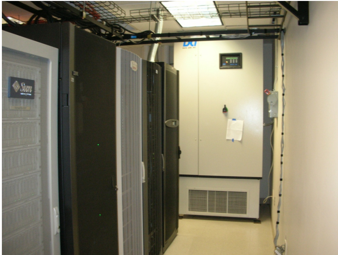
Shows Servers and 1 of the 3 new 11-Ton Air Handler Units
