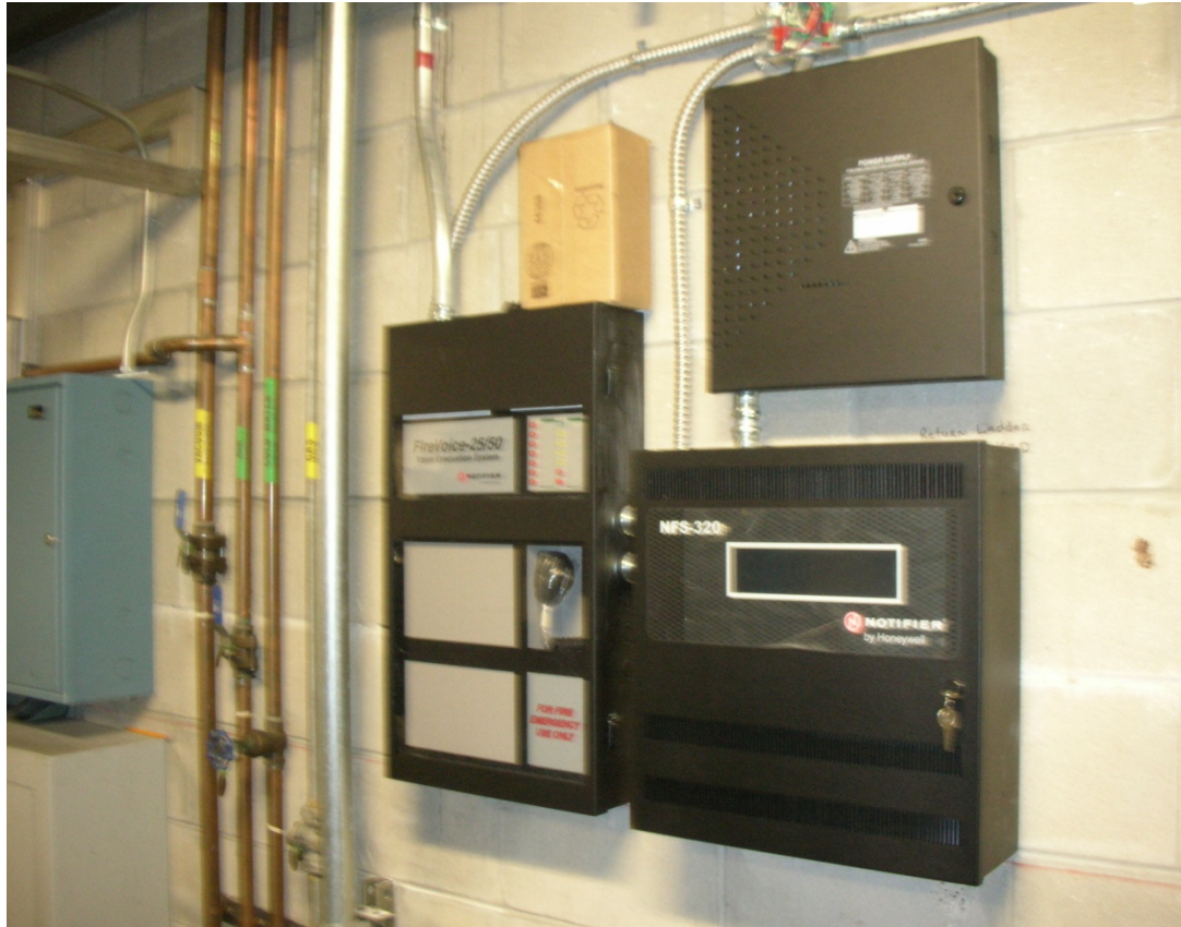
Picture of New Fire Alarm Panels
